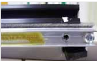
The plastic guide protruding out the bottom of the sliding sash
